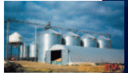
Installations of loop systems with existing bins.
